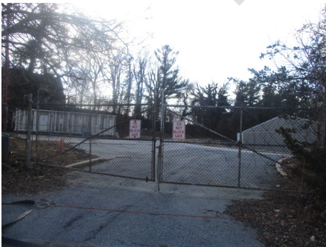
RESTRICTED ACCESS TO COMM. TOWER
