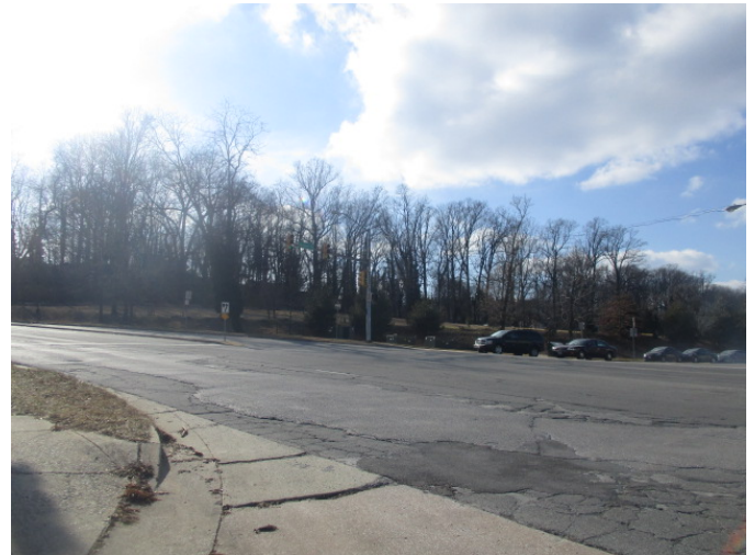
CURB-CUT FROM BOSLEY AVE.
